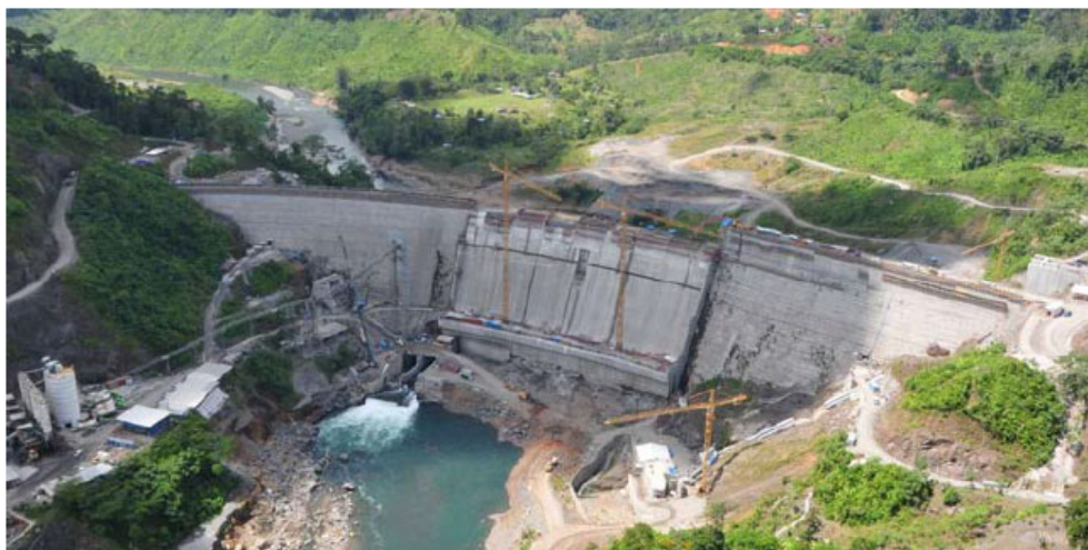
Changuinola Dam H=105m, L=600m
