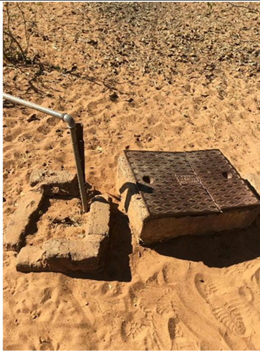
Figure 9.25 Piped Water in the Project Area
