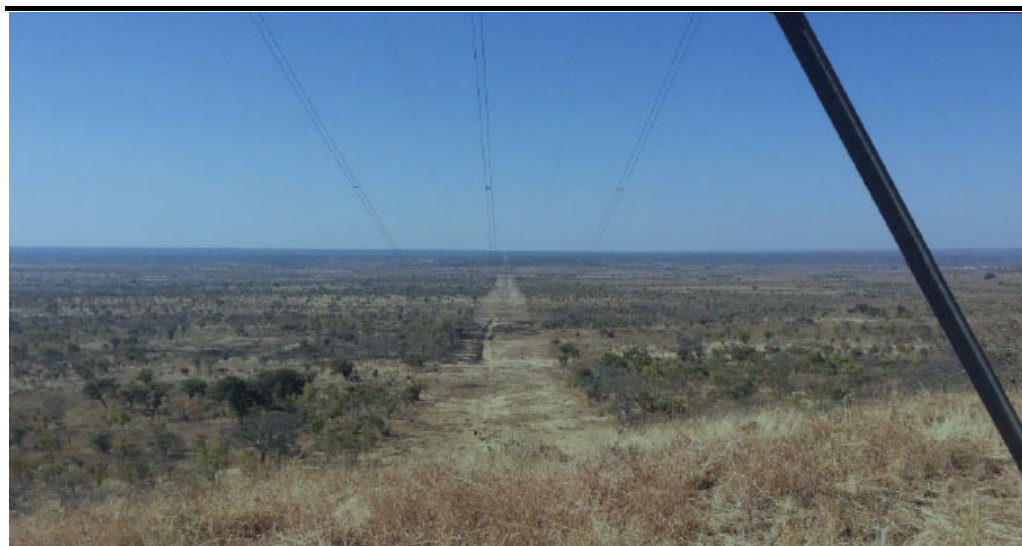
Figure 2.8 View of the RoW of Mukuni-Muzuma 330kV Transmission Line
