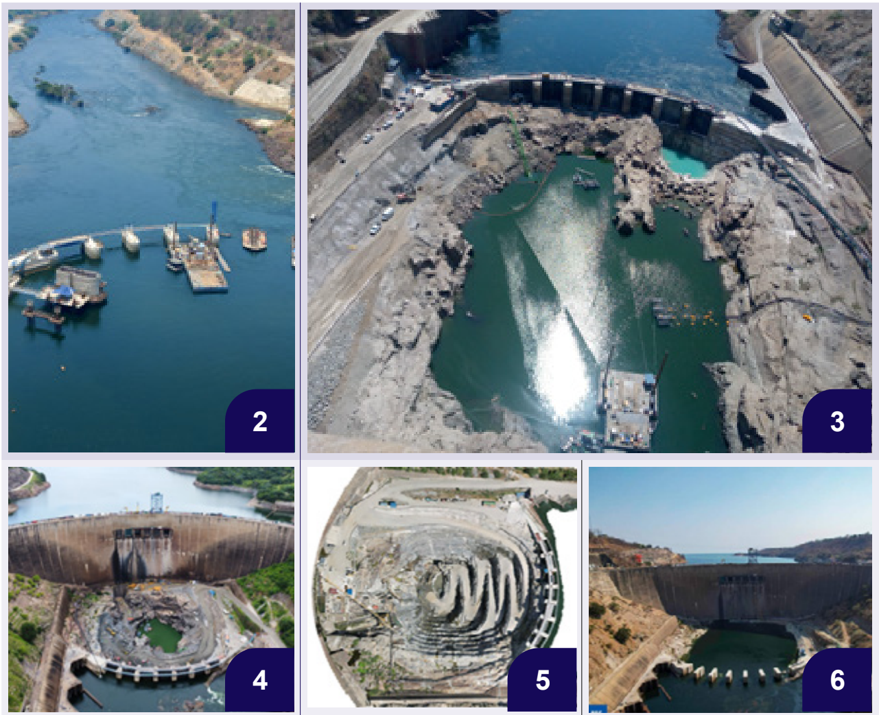
Figure 30 - The progression of Plunge Pool Works from commencement to completion
