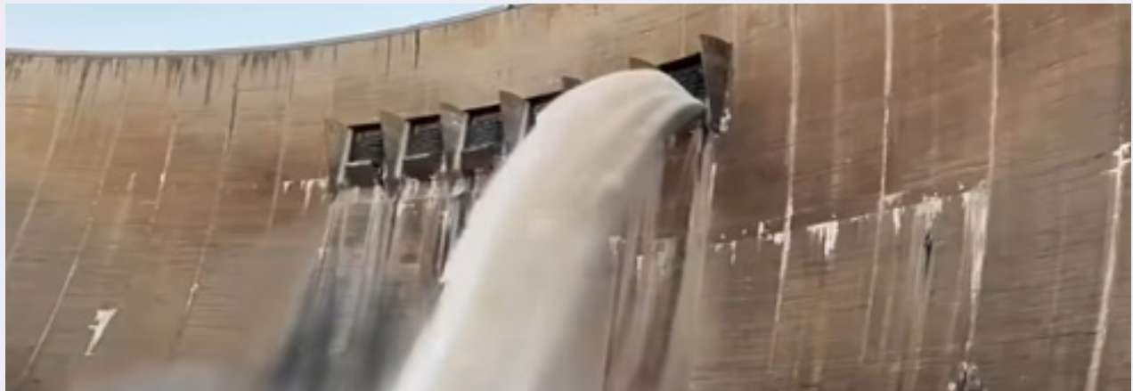
Figure 32: Sluice 6 leakage testing.
