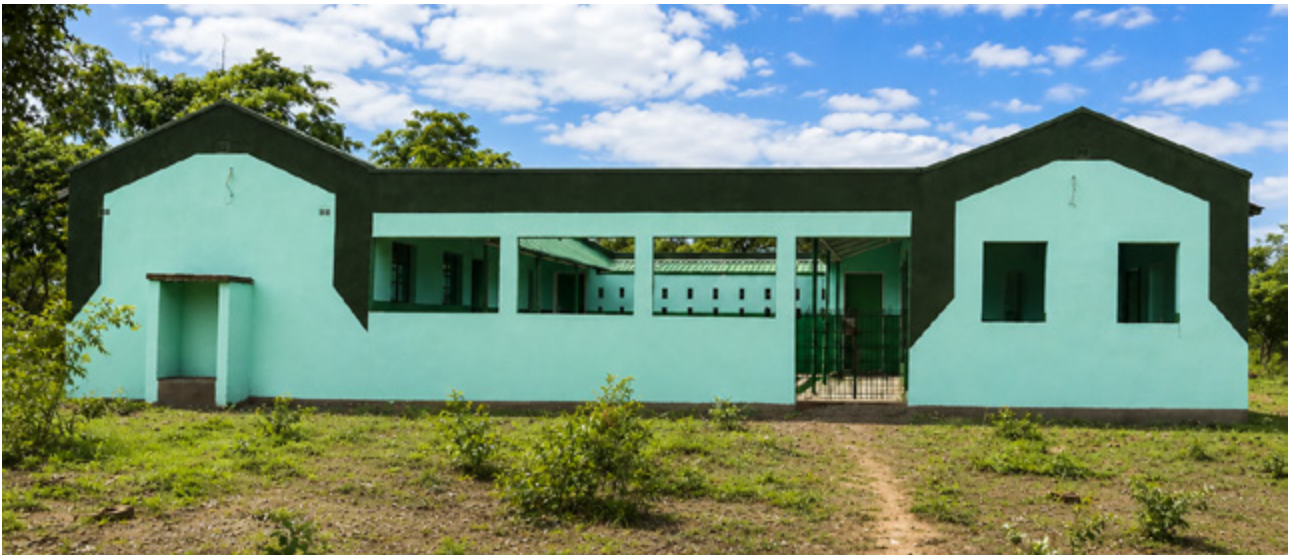
Chidyamugwamu Rural Health Centre under construction in Zimbabwe.
