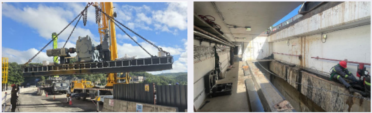
Figure 33...Spillway Hoist installation
