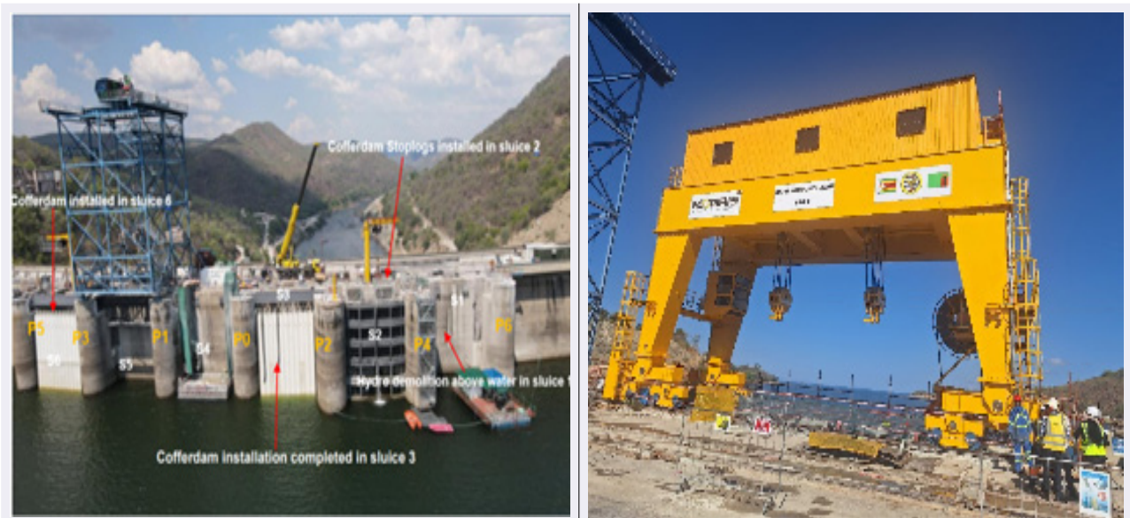
Figure 31: Works layout and Gantry Crane partial hot commissioning
