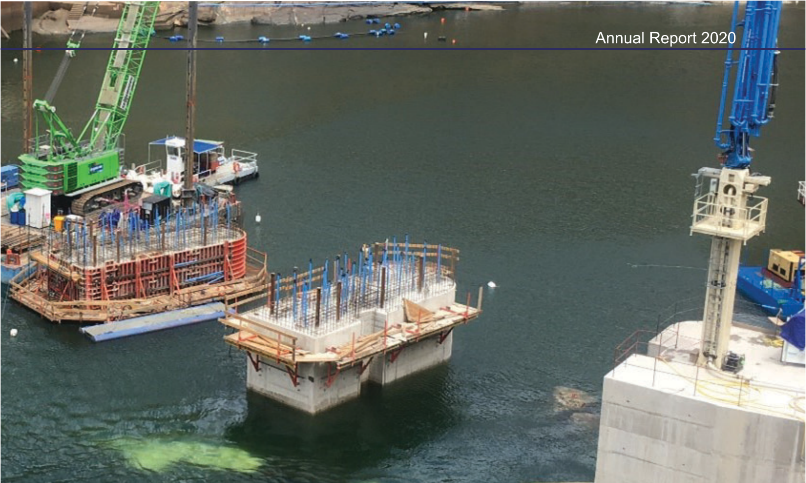
KDRP Plunge Pool reshaping Cofferdam Piers under construction
